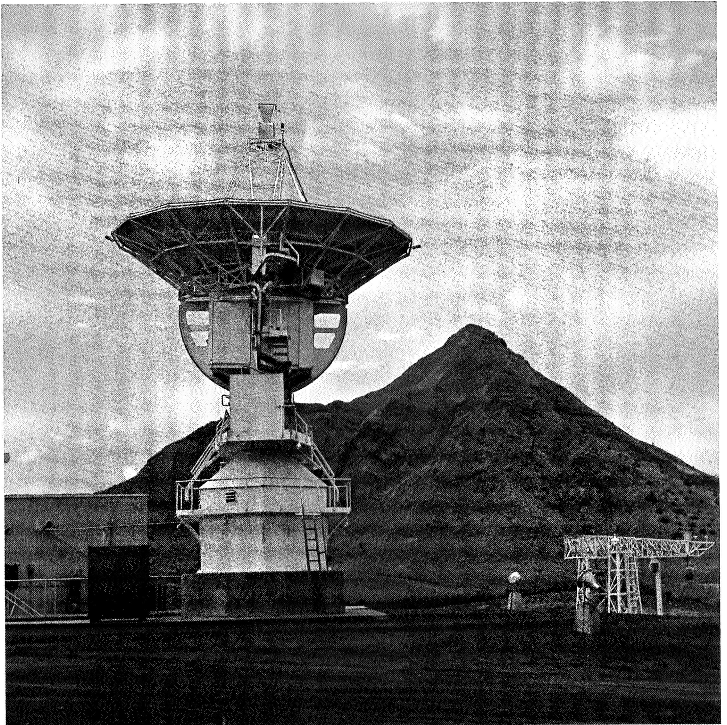
The DSIF antenna at Ascension Island, which has a 30-foot-diameter paraboloidal reflector mounted on an azimuth-elevation axis system, is capable of high angular velocities and accelerations to track a "close in" spacecraft.
